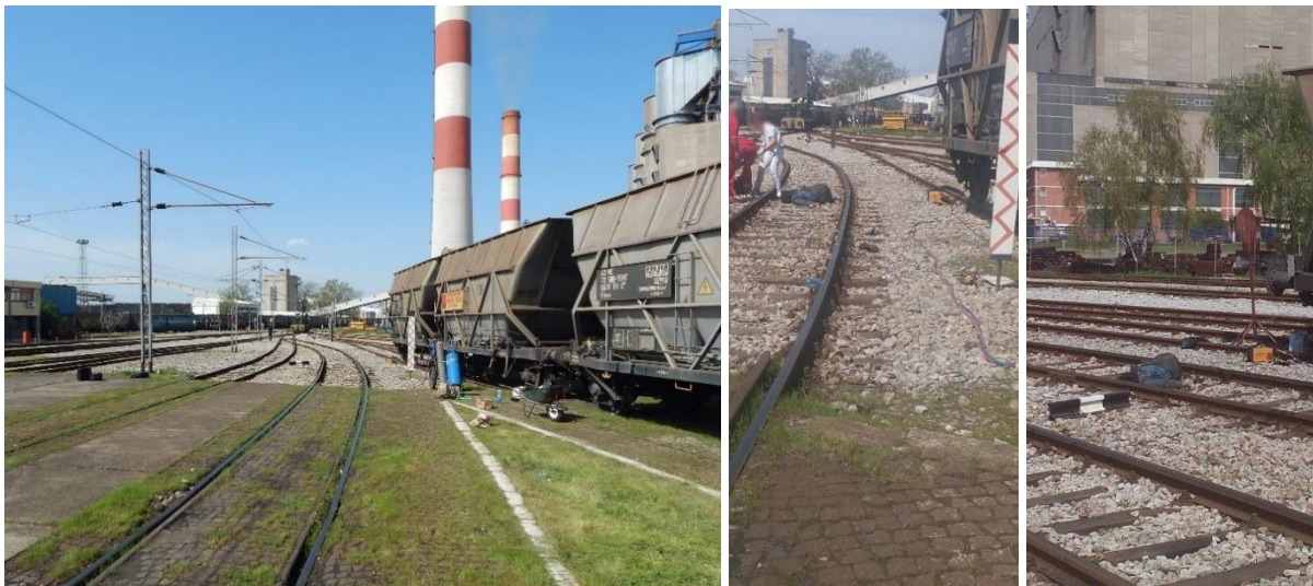
Fig. 4.2.1.1: The appearance of the site where it came to overtaking of the locomotive CEM-7 on the worker
