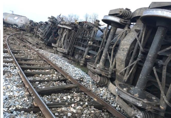
Fig. 3.7.2: Appearance of derailed wagon
