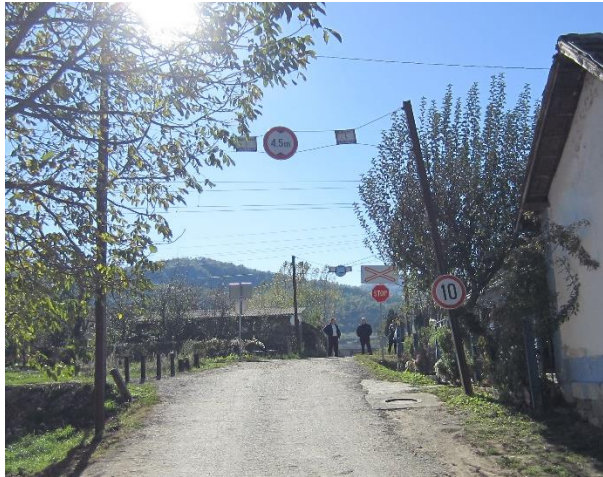
Fig. 3.5.1: Appearance of level crossing (viewed from the direction of center of Grdelica)
