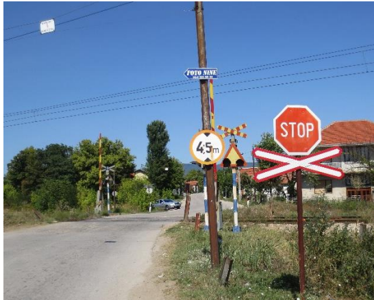
Fig. 3.3.1: Appearance of level crossing (from the direction of the settlement Kutleš)
