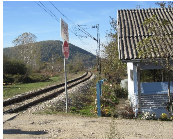
Figure 4.4.1.2: Appearance of the facility – the guard
