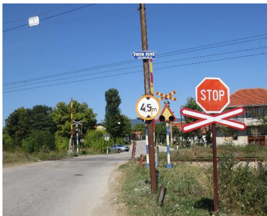
Figure 4.2.1.1: The appearance of the crossing (from the direction of the settlement Kutleš)
